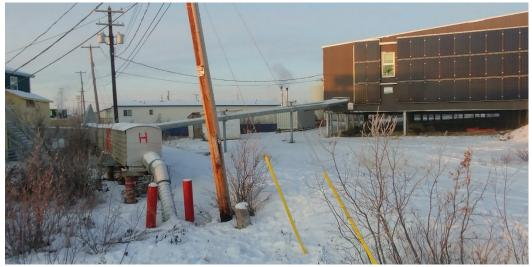
Figure 5. Utilidor located to the north of site option B (north of Arctic Store)
