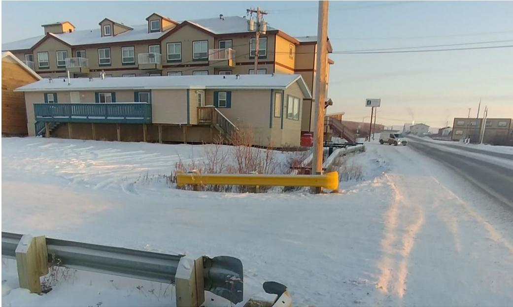
**Figure 3. Utilidor seen routing down and below access road to church parking area**
